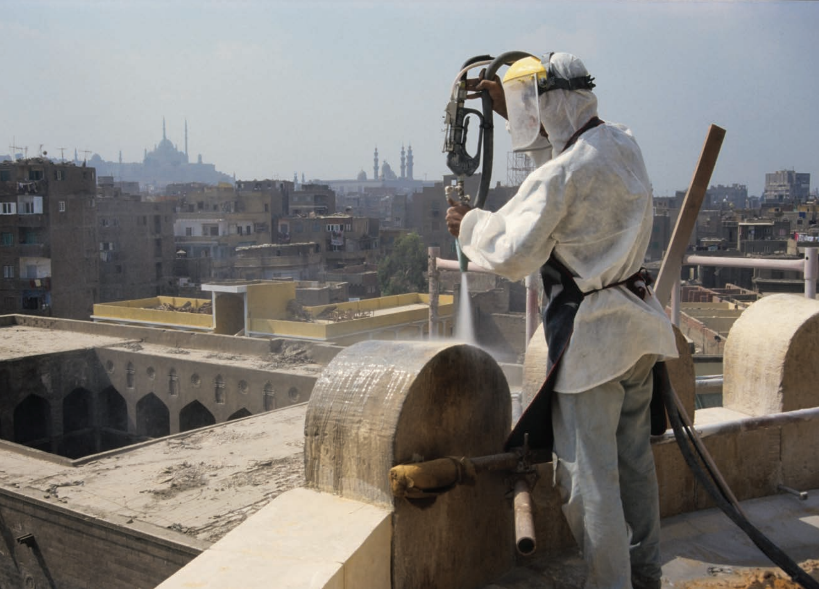
A technician cleans Bab Zuwayla with a pressurized water jet. The Citadel is visible in the distance.
