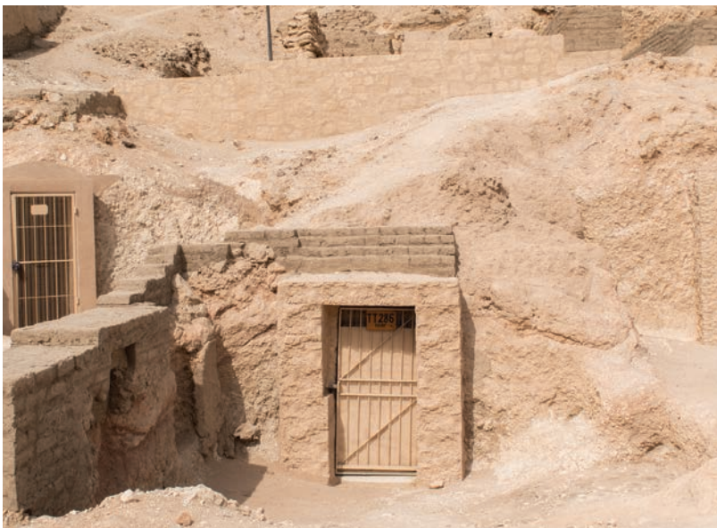
Top: The facade of TT286 before ARCE's interventions
