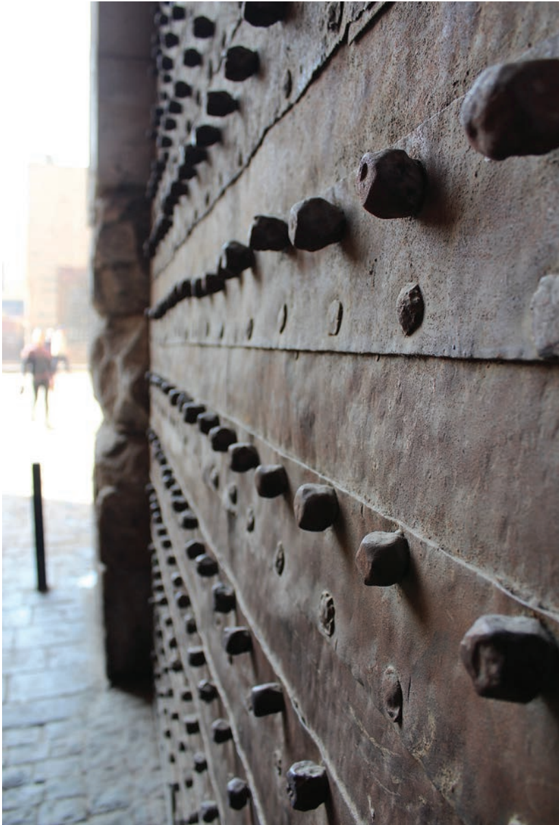
A close-up of the large iron nails that protrude from Bab Zuwayla. Photographed in 2019.
