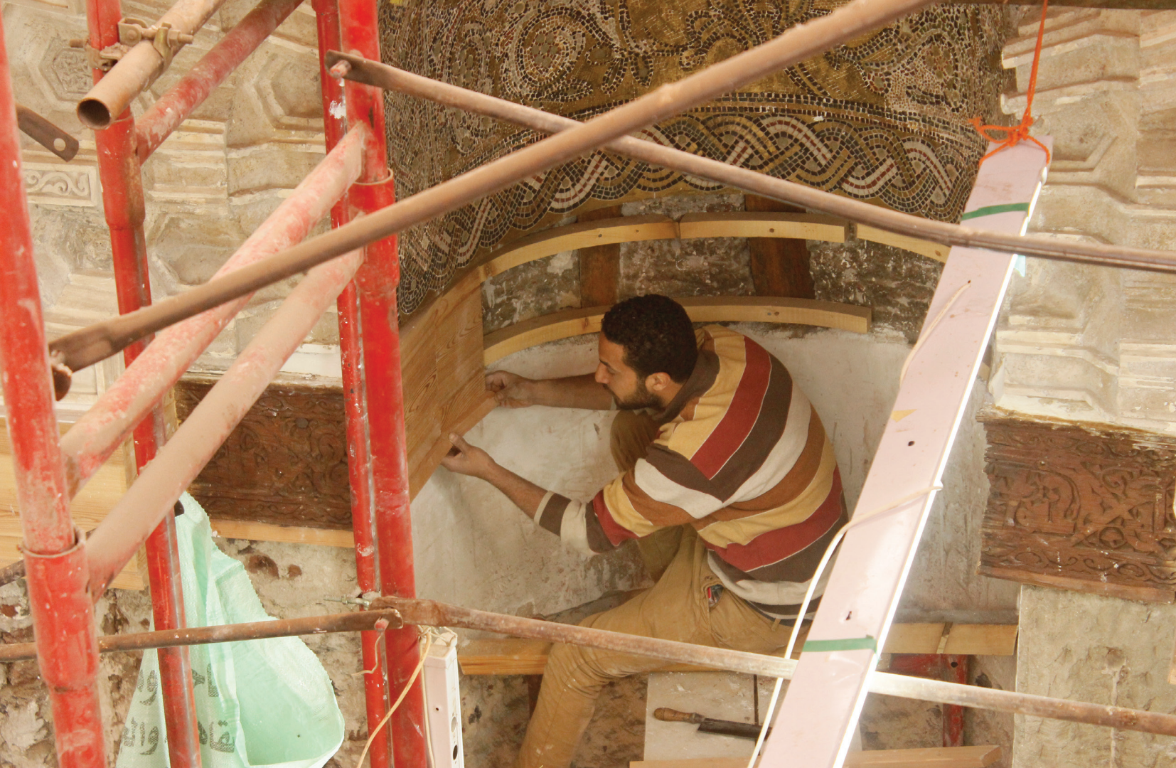
Top: Carpentry work on the lower frieze
